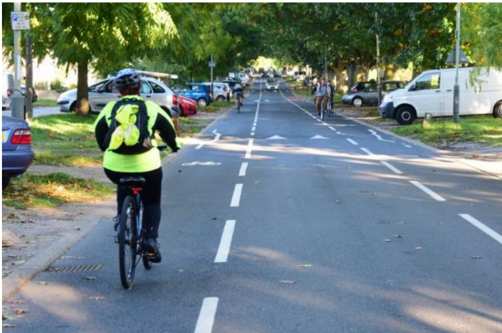
Figure 13: The Avenue, Norwich, with centre-line removed and kerb-side cycle lane instead
