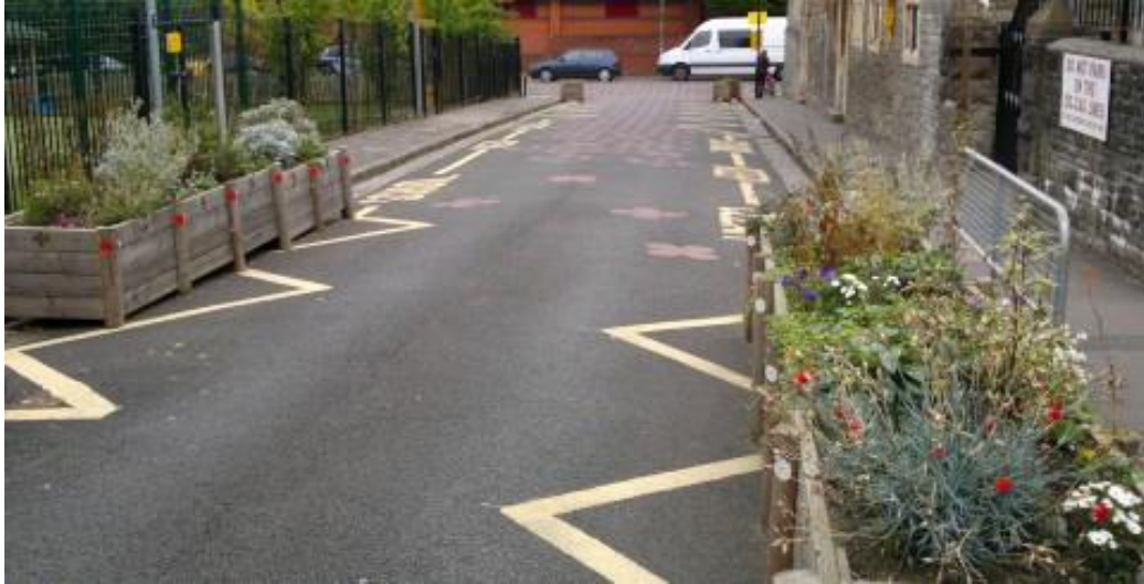
Figure 10: Planters placed in carriageway to discourage stopping outside school and reduce speed
